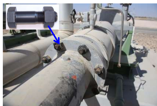
Fig.4 Nuts & Bolts reinforced by CNT paint in oil field in middle east country
